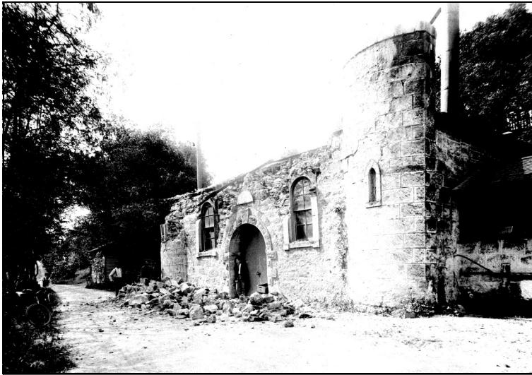
Beringer Distillery Building. Courtesy Beringer Family Collection
